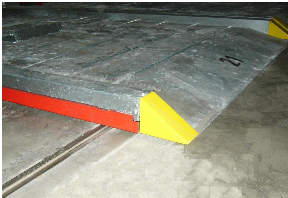
Platform with end cap, ramp, guide rail, safety bar
